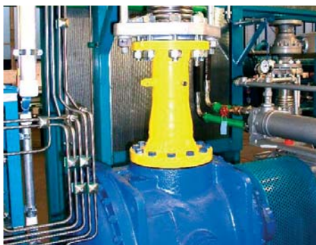
Gas Turbine Installation
